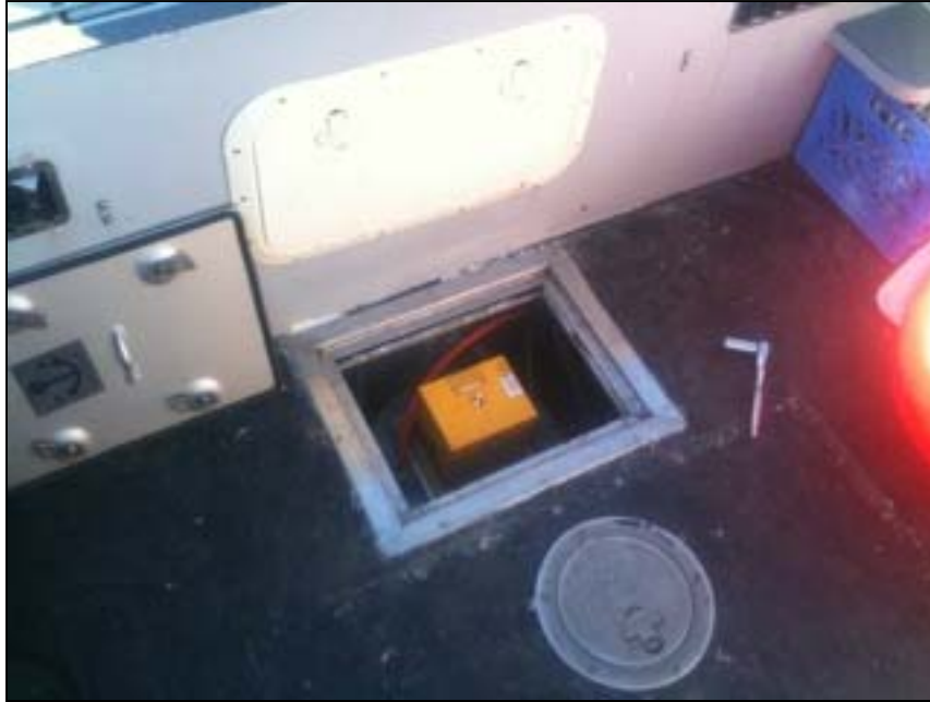
Figure 3: IMU Installation, POS M/V 320 V4 IMU shown. 2014 season utilized POS M/V 320 V5 IMU.
