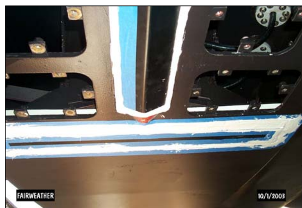
Figure 4: Installed on Fairweather
