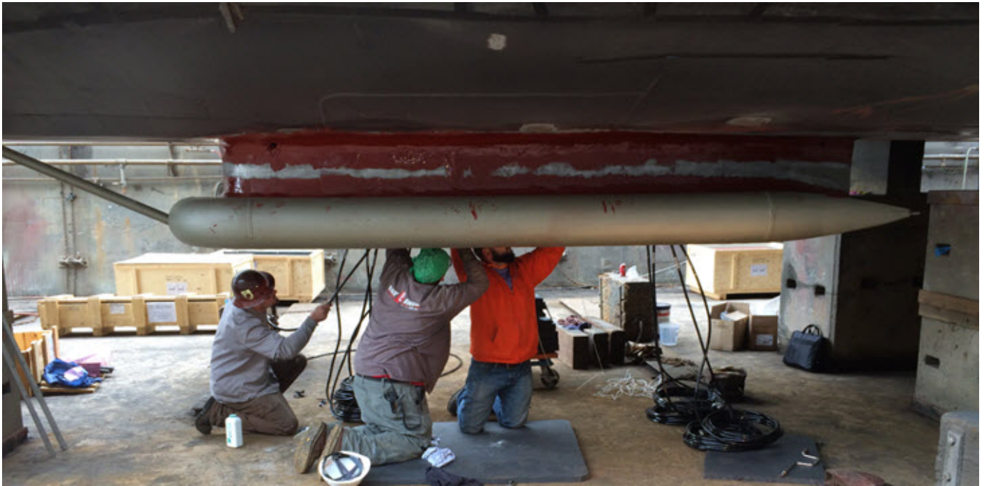
Figure 13: EM 710 Gondola during transducer installation.
