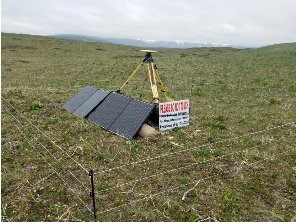
Figure 4 – Project GPS base station installed on the Ikatan Peninsula.
