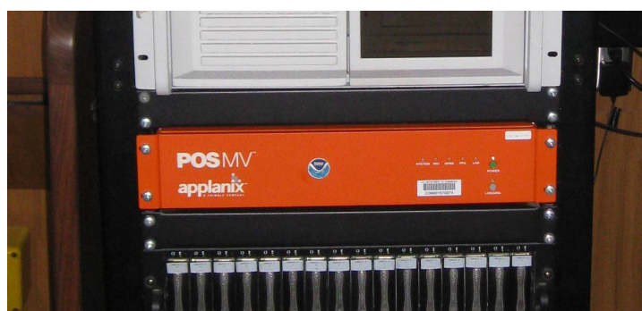
Figure 6: POS MV Topside Unit
