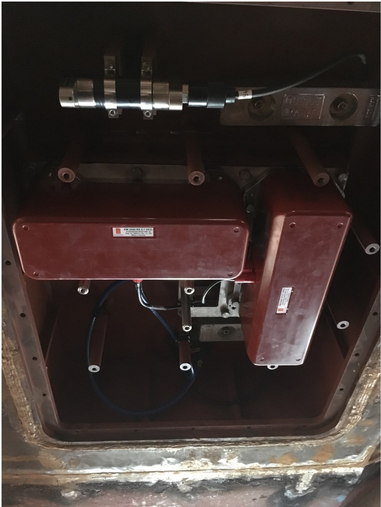
Figure 3: The EM2040 system mounted on the hull of R352, shown during initial installation in 2018.
