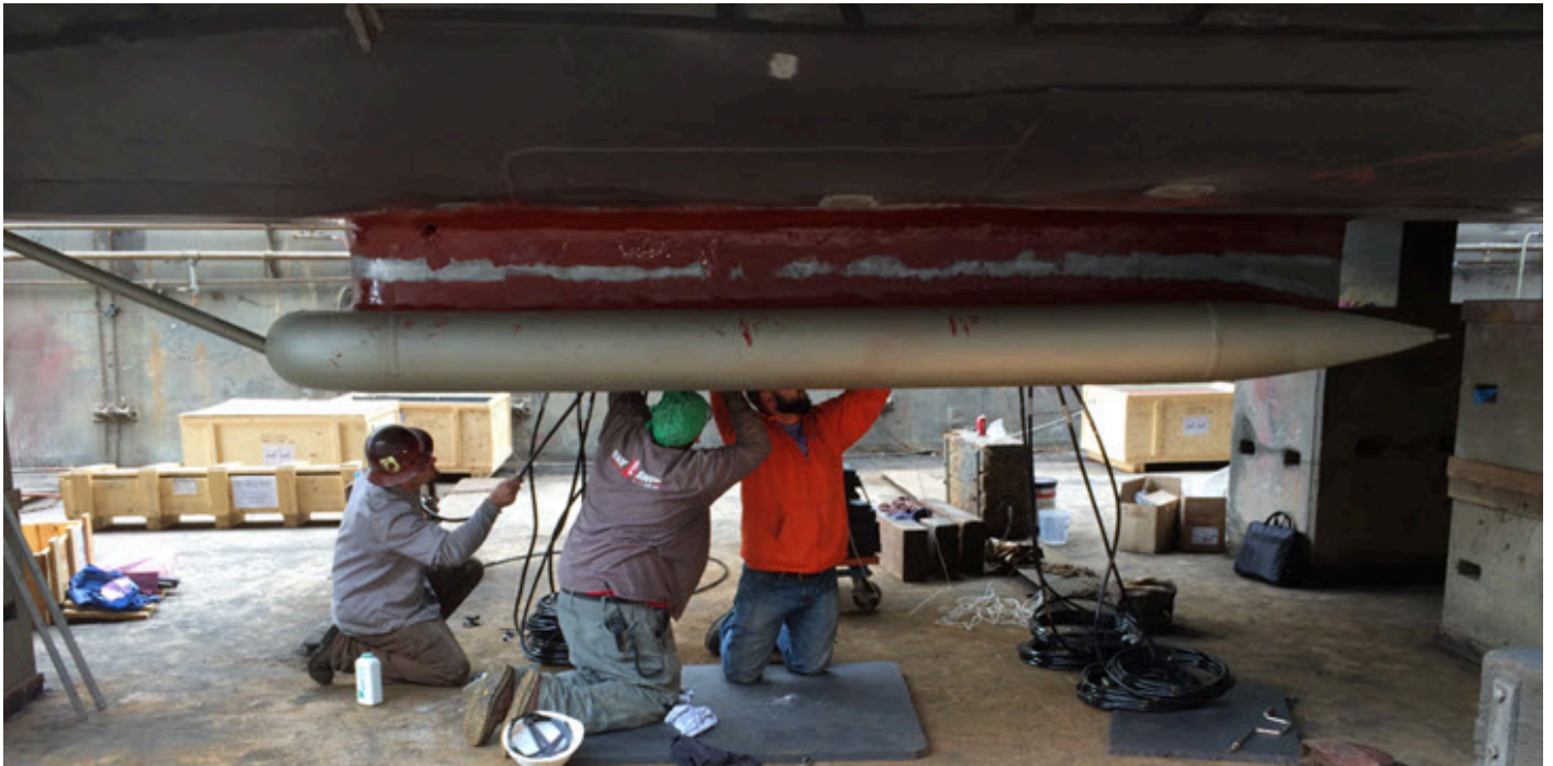
Figure 6: EM 710 gondola during transducer installation
