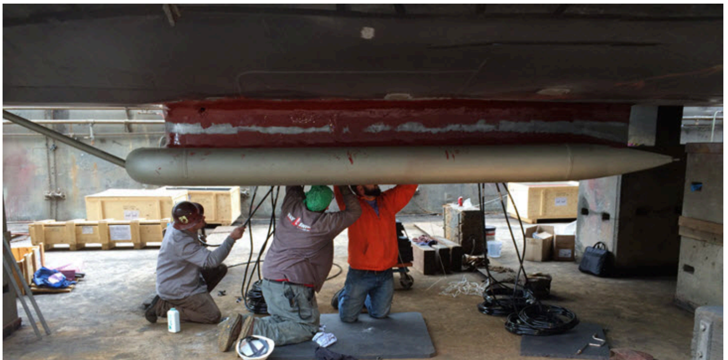
Figure 2: EM 710 gondola during transducer installation
