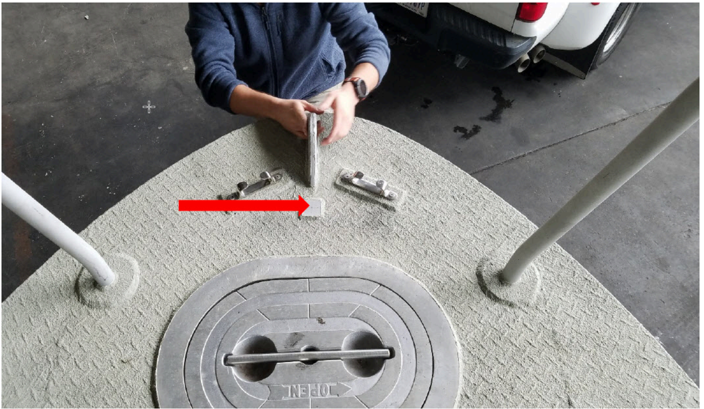
Figure 19: Benchmark location, centerline forward on S3006
