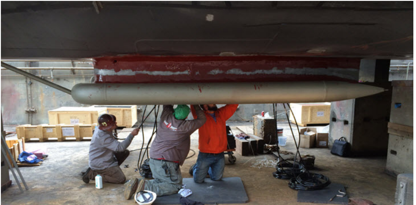
Figure 8: EM 710 Gondola during transducer installation.
