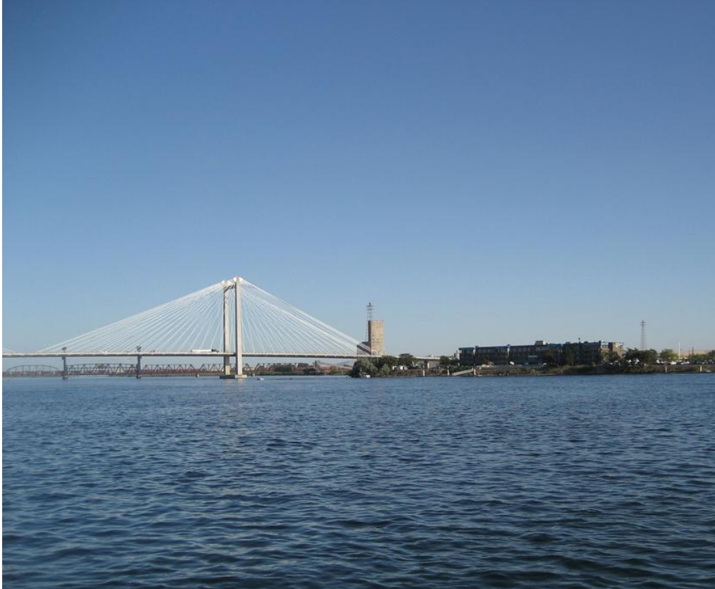
Clover Island and Benton-Franklin Intercounty Bridge
