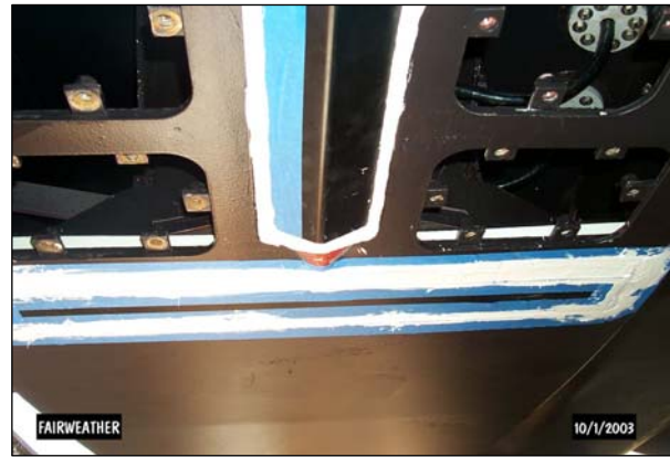
Figure 4: 8160 Installed on Fairweather
