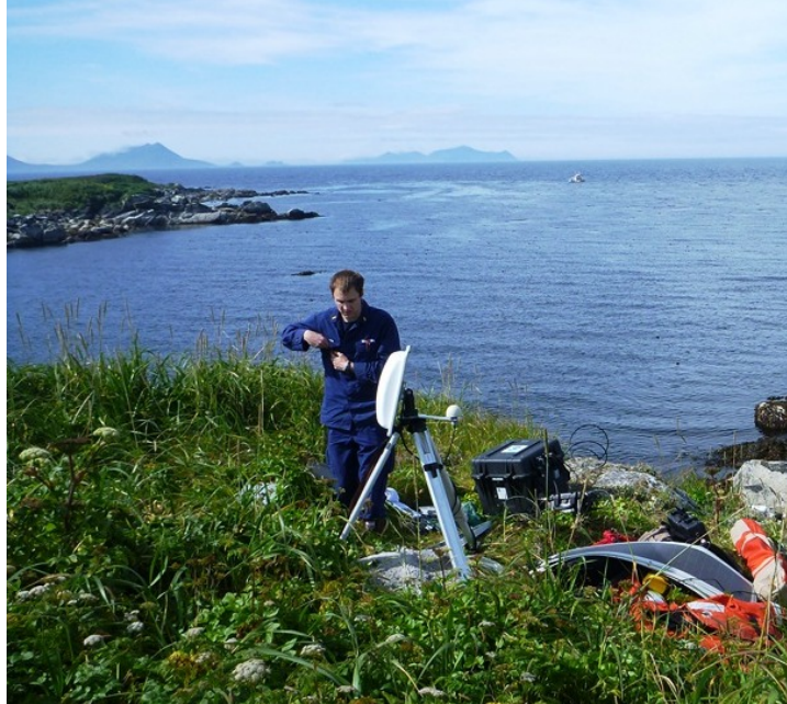
Figure 22: A Portable Tide Gauge (PTG) system with GOES and GPS antennae mounted on a aluminum tripod. Unsecured orifice tubing can be seen heading towards the water.
