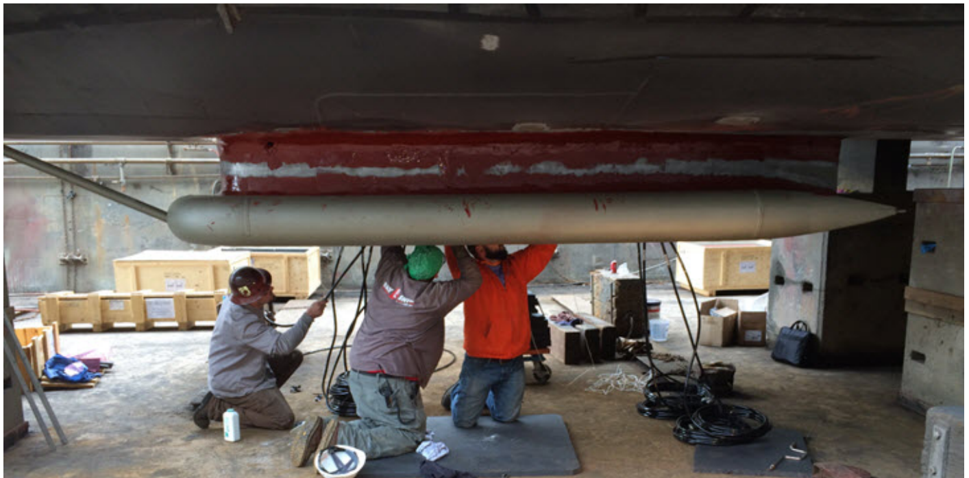
Figure : EM 710 Gondola during transducer installation.
