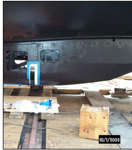
Figure 2: 7111 Installed on Fairweather
