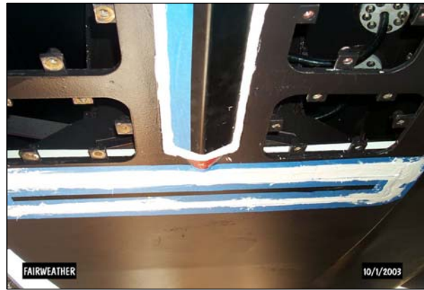
Figure 4: 8160 Installed on Fairweather
