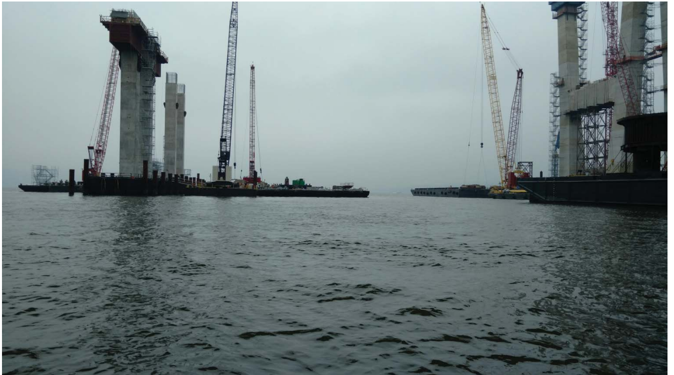
Figure 2. Barges rafted to bridge pier.
