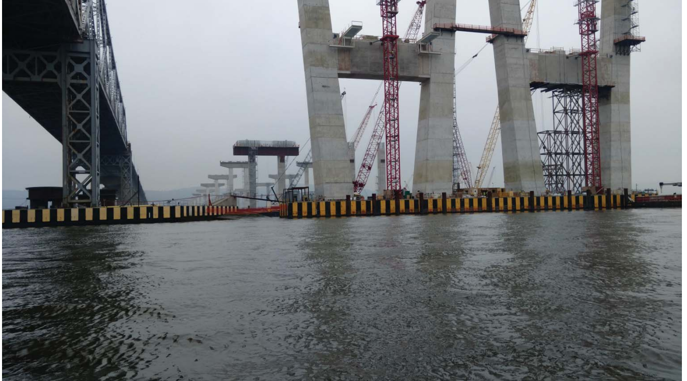
Figure 1. Overview of current Tappan Zee Bridge with new bridge piers under construction nearby.
