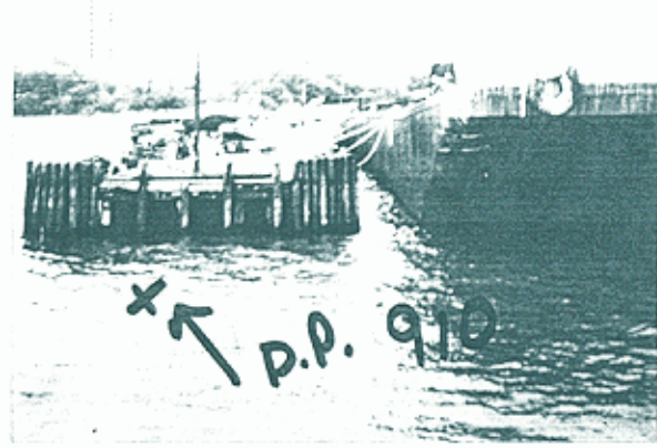
WOODEN TUG & BARGE PIER D.P. # 910 DISTANCE: 12M θ: 075°T
