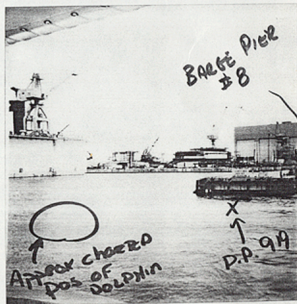
BARGE PIER #8 CHARTED CHARTED DOLPHIN DOES NOT EXIST D.P. 919 \Theta: 067^{\circ}T DISTANCE: 13M
