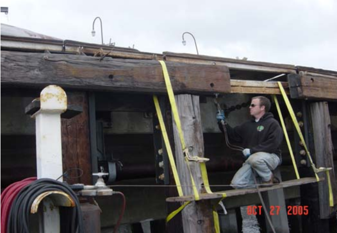
Photo No. 1 Burning off the old bolst from the whaler
