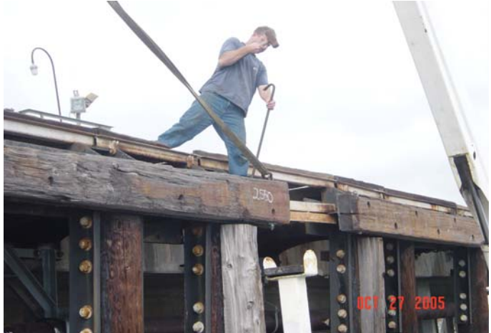
Photo No. 3 Using the Boat Crane, the old whaler section was removed.
