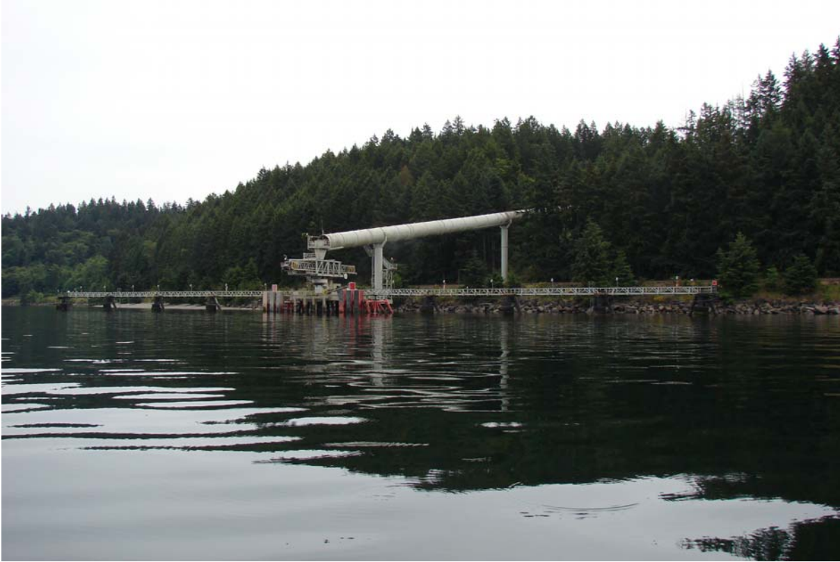
Photos taken by the NRT3 of the uncharted pier:
