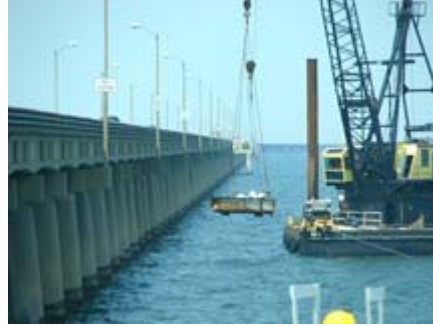
Rip Rap Stone Being Placed with a "Skid Pan"
