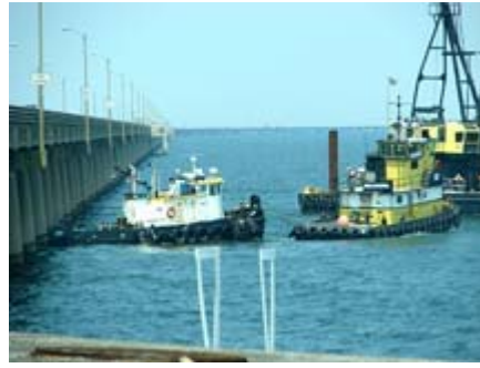
Tugs Position the Rig Prior to Stone Placement
