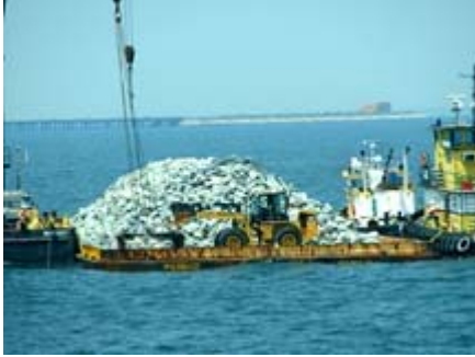
Front End Loader Filling the "Skid Pan"
