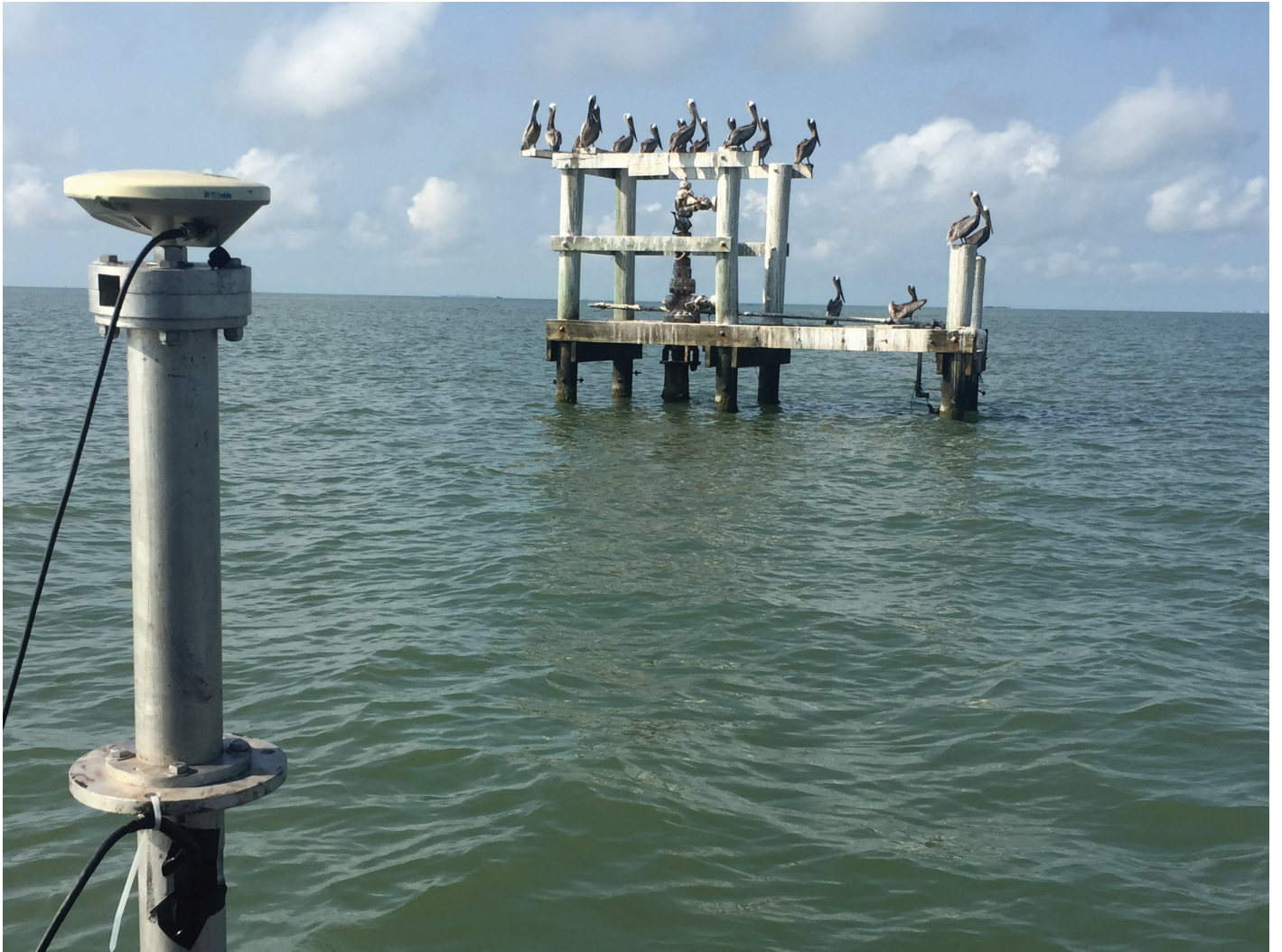
Figure 18: Uncharted obstruction (wellhead) submitted as a DTON
