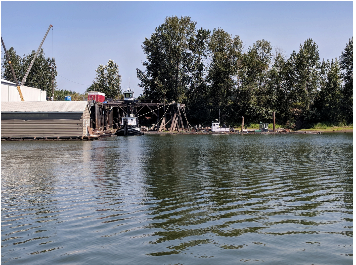
Figure 4: Various examples of vessels, ruins, and barges blocking the shoreline in the southeastern portion of Swan Island Basin.
