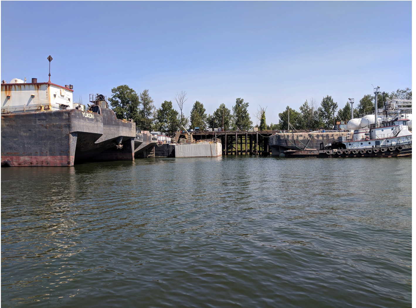
Figure 6: Various examples of vessels, ruins, and barges blocking the shoreline in the middle of the survey area on the eastern shore of Swan Island Basin.
