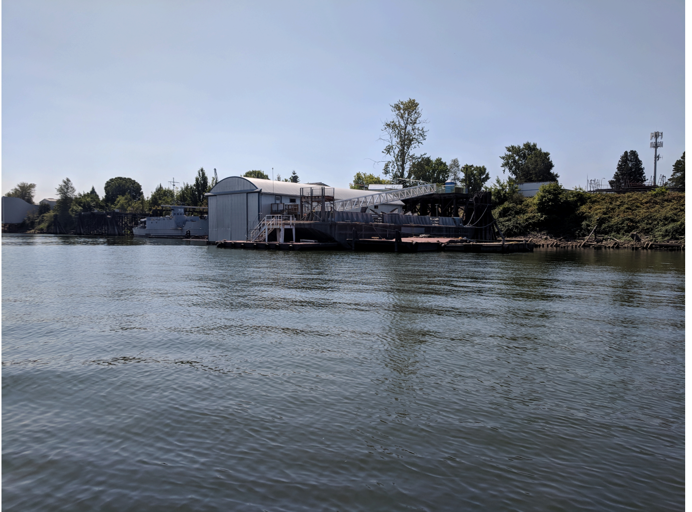
Figure 5: Various examples of vessels, ruins, and barges blocking the shoreline in the southwestern portion of Swan Island Basin.
