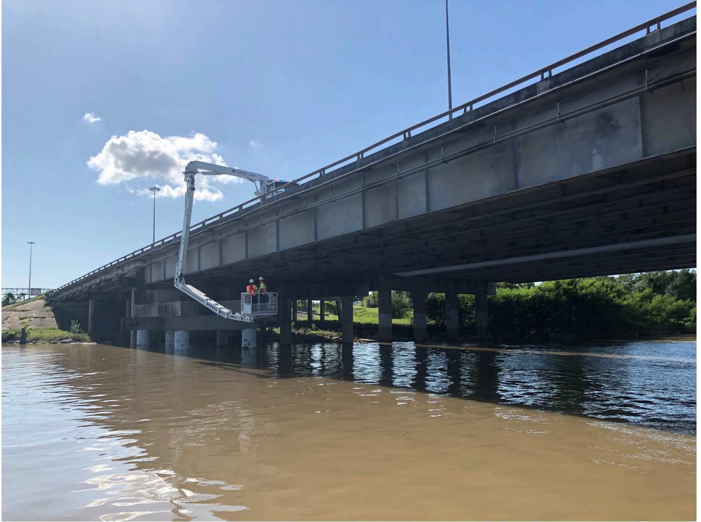
Figure 16: Department of Transportation Inspectors, Interstate 10 Bridge, Westbound Segment. Picture facing Southeast.
