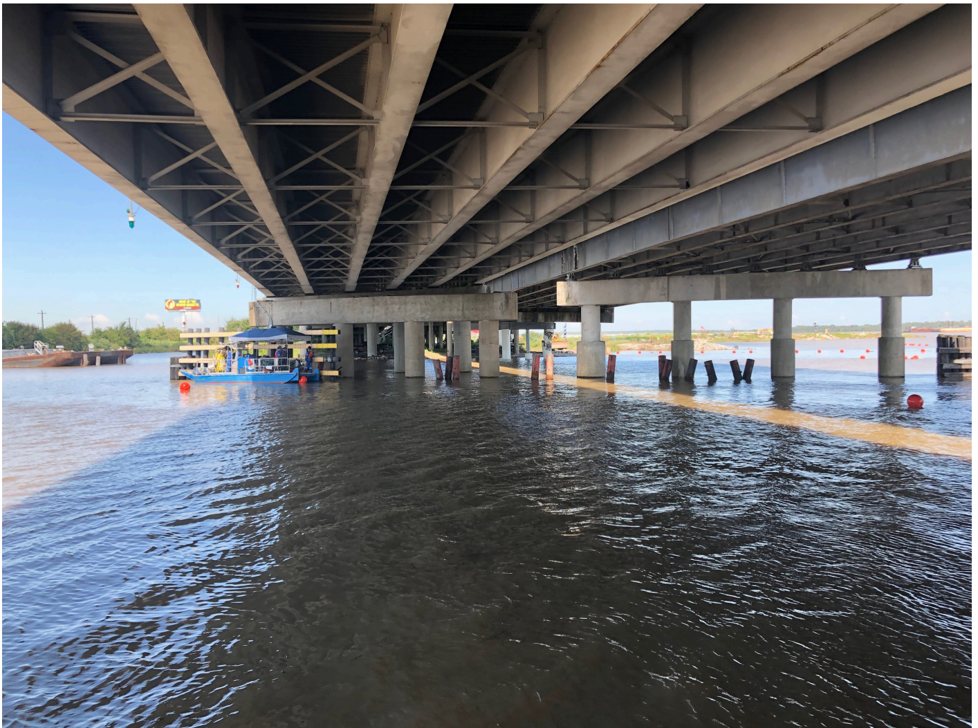
Figure 11: Maintenance Crew Remedies Detached Fender Fence. Picture is facing west.
