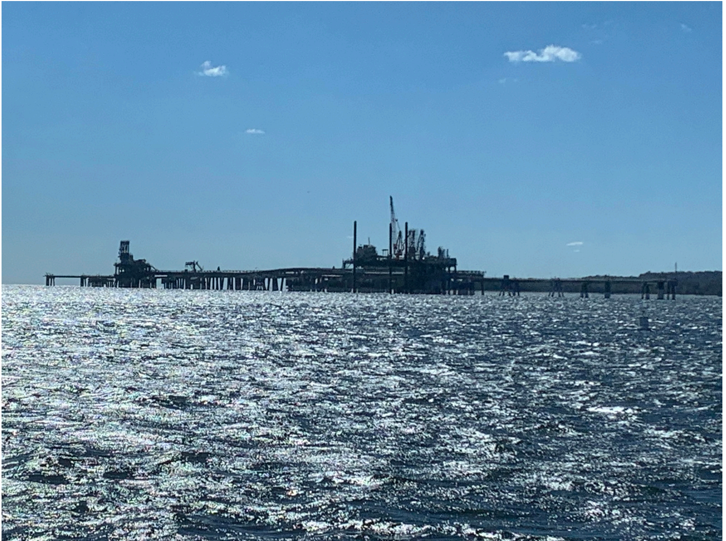
Figure 17: Cove Point LNG Terminal platform.
