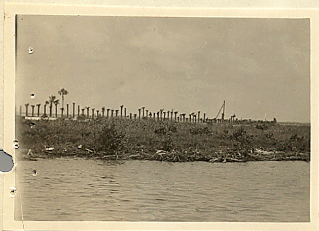
NEW BULKHEAD AT BARRONS RIVER
