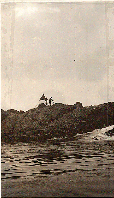
UNALGA ISLAND: Topographic signal (tripod) JUMP on a 12 foot lava islet about 1/4 mile east of the main island. View looking to the south.
