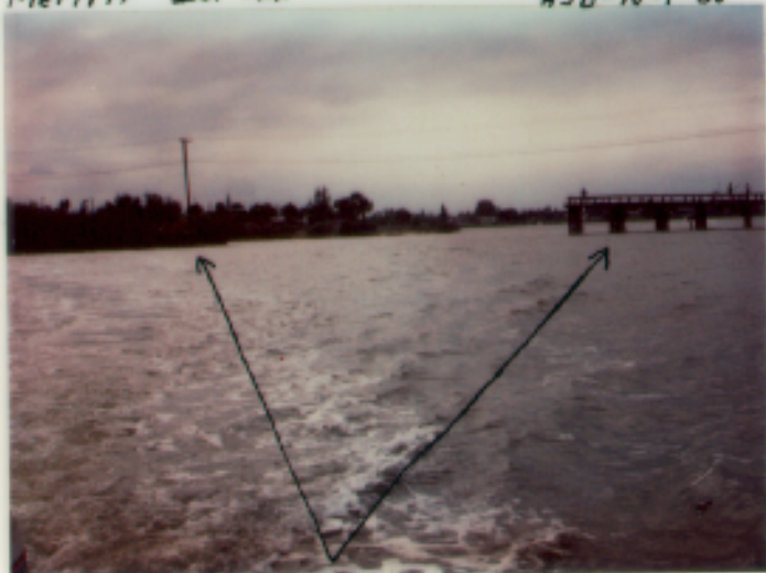
Bridge in Ruins on Audubon Rd. on Sykes Creek
