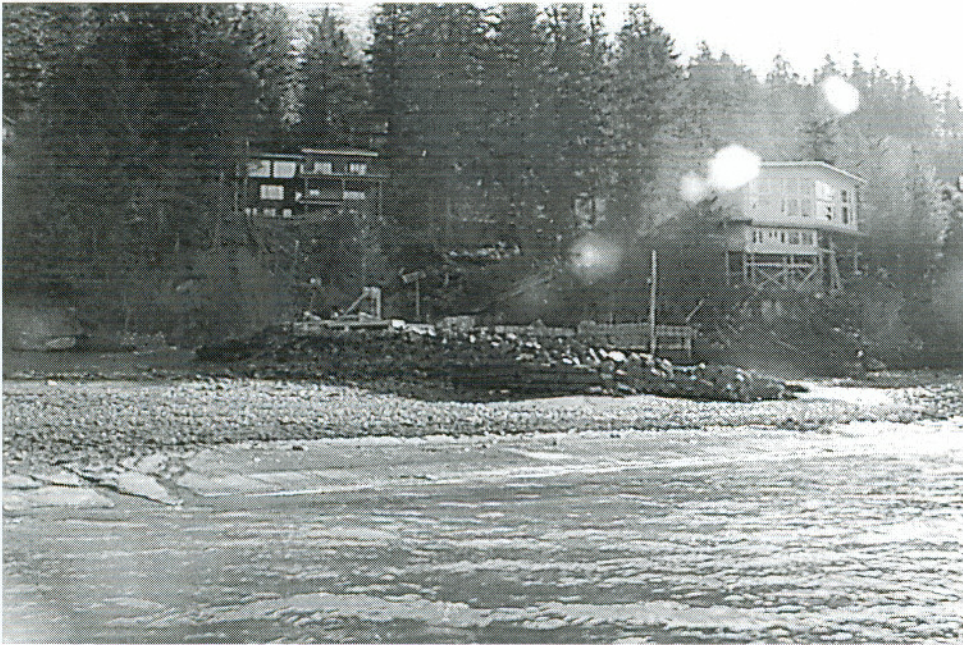
Figure 3: Fix 40830, RIPRAP BREAKWATER/BOAT RAMP-PRIVATELY MAINTAINED LAT. 58:15:12.046N, LONG. 134:18:48.247 W ✓
