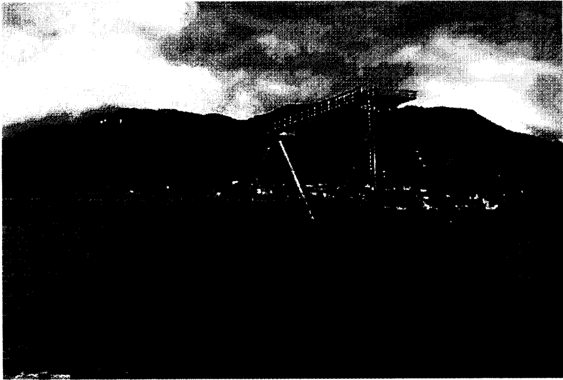
Photo 3. New north catwalk – part of new modifications to Haines City Pier
