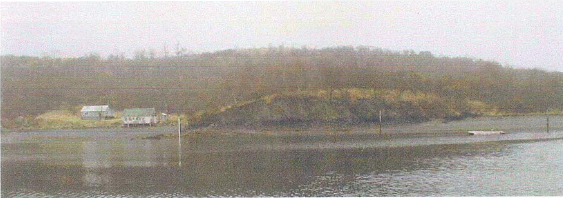
PHOTO: 20000–20004 piles floating dock AW 51743
