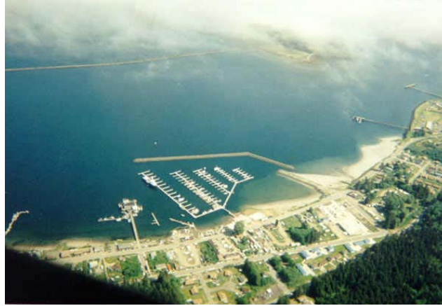
Figure 2. 1997 Aerial photograph of Makah Marina
