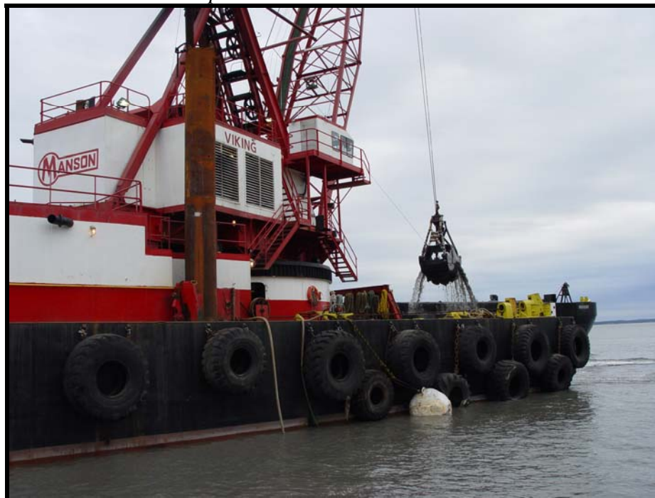
Manson Dredging Operation at the Port of Anchorage
