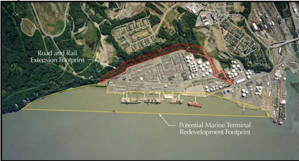
Aerial Overview of POA Intermodal Expansion Project
