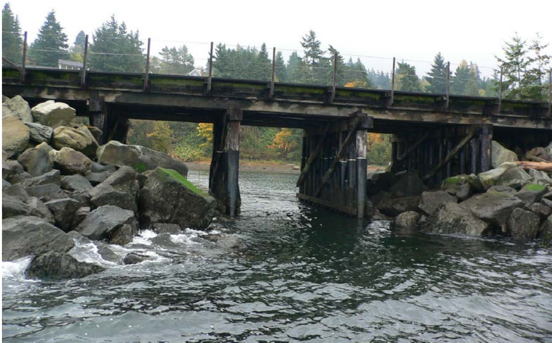
Figure 10: Image of railroad causeway just south of Post Point
