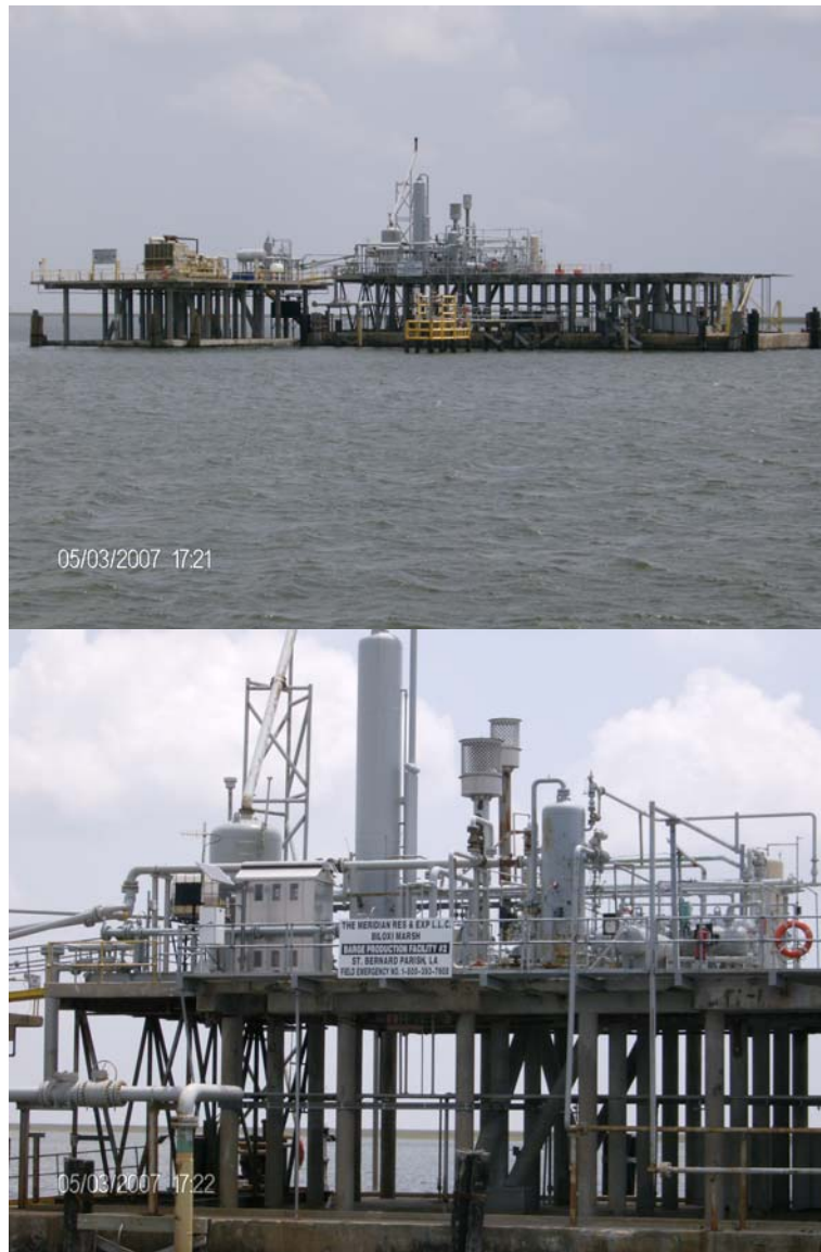
Figure 1 Photographs of Platform within H11613 in 30° 00' 43.299"N 089° 32' 39.608"W (NAD 83).
