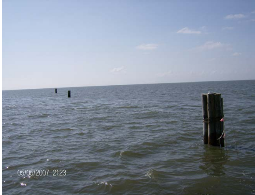
Figure 26 Photograph of Dolphins Exposed Approximately 8 feet (2.4 meters) above Chart Datum within H11613.
