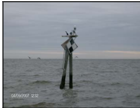
Figure D-10. Day Beacon at Proctor Point
