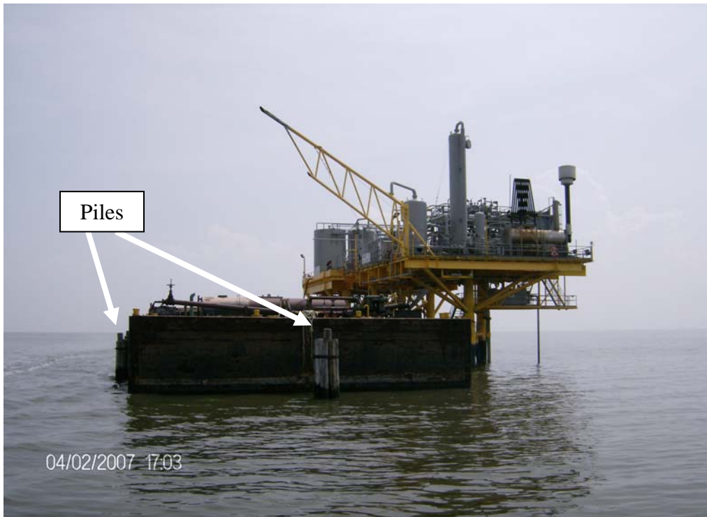
Figure V-11 Photograph of barge moored to piles by MANTI A and B within H11615.
