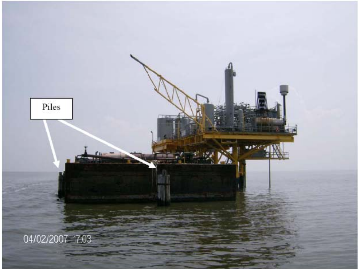
Figure 2 Photograph of barge moored to piles by MANTI A and B within H11615.
