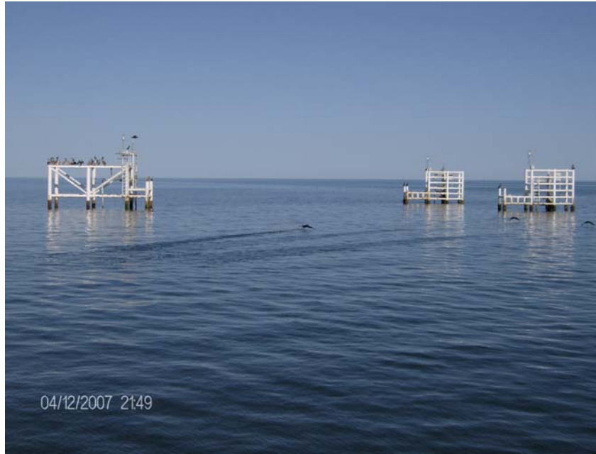
Figure V-16 Photograph of Three Platforms within H11615.
