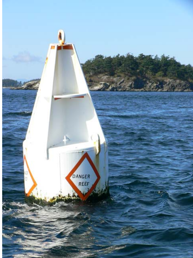
Figure 12: Clements Reef Danger Buoy (Light List # 19860). Note the absence of a topmark.
