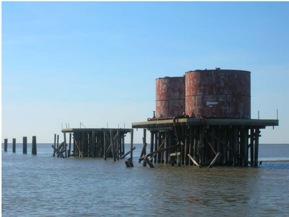
There are twenty-one piles surrounding a barge terminal area.
