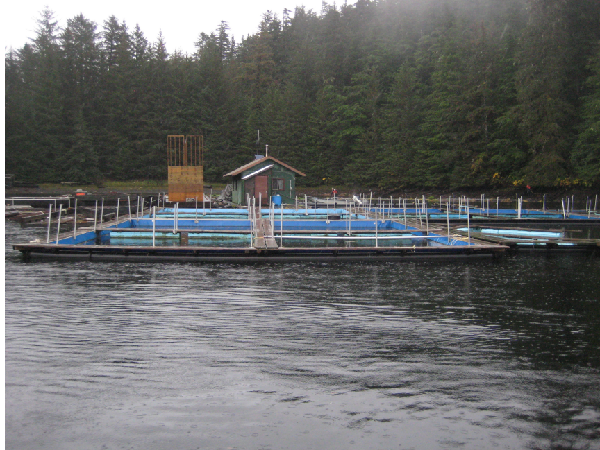
Figure 43: New fish pen located in Little Port Walter
