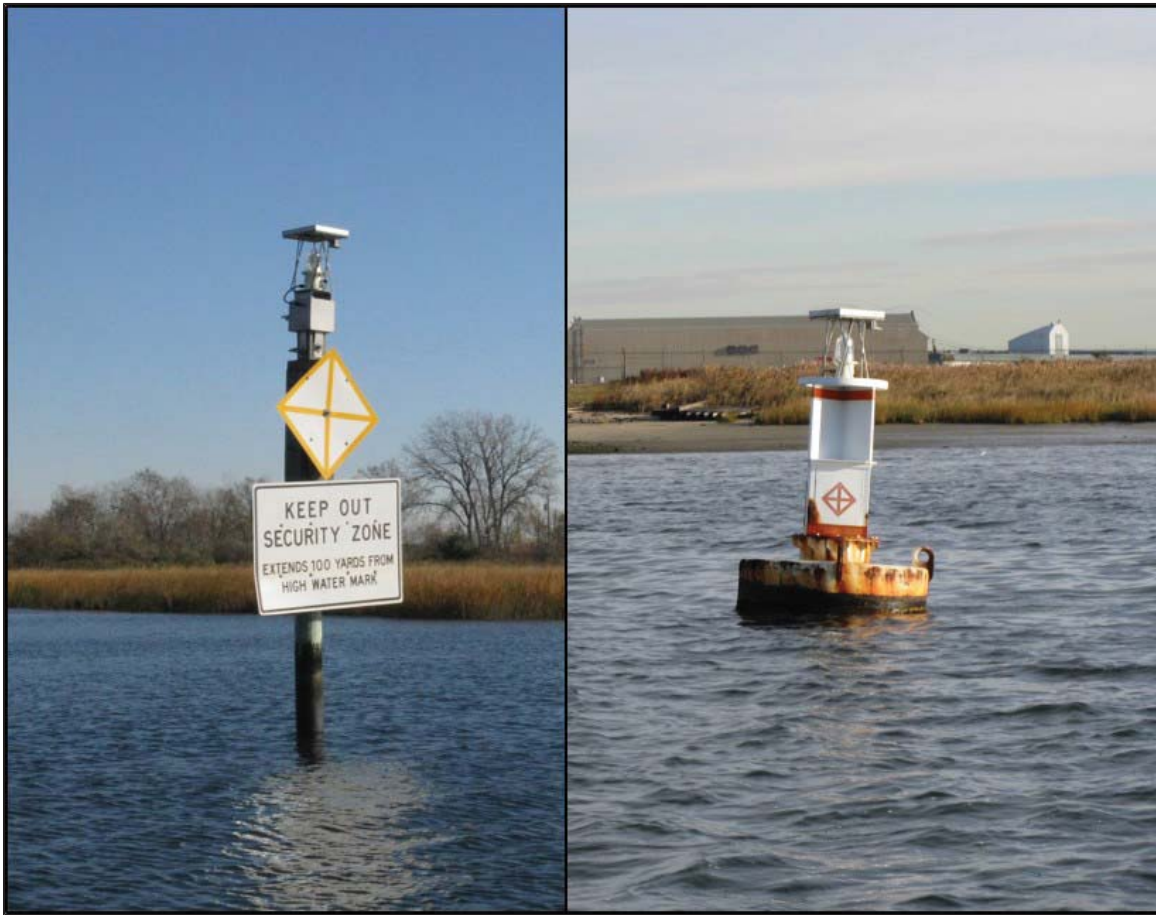
Figure 42: Photos of typical fixed and floating JFK security zone aids to navigation.
