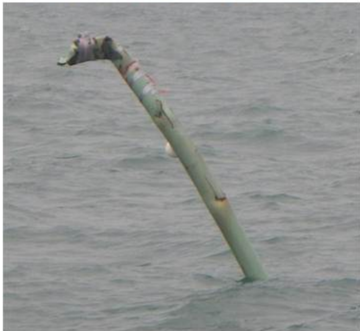
Exposed Pipeline close to pipeline position from LA DMR data. Position from Sonarwiz - Lat: 29°50.37827'N Long: 88°57.01320W
