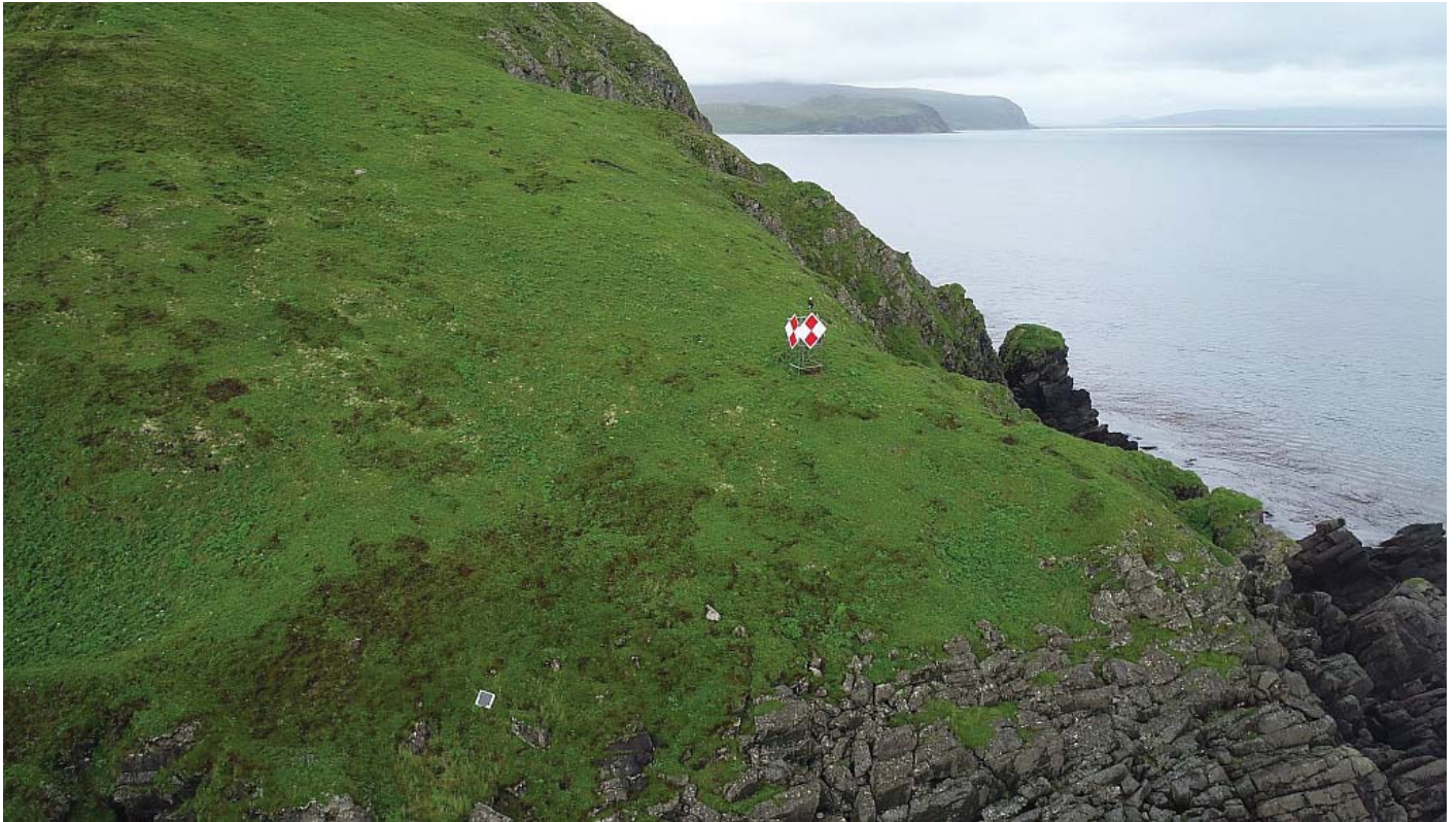
Figure 16: Ikatan Point Light ATON during this survey
