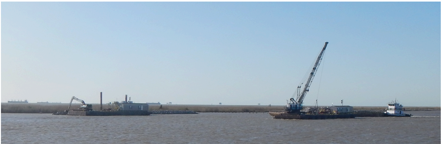
Figure 32: Ongoing construction observed during H13212 survey operations
