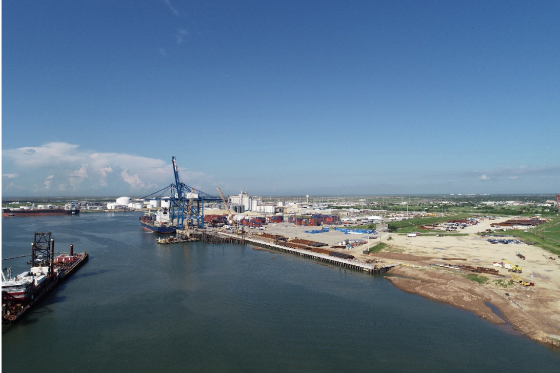
Figure 38: Active Construction at Port of Freeport, Photo 1
