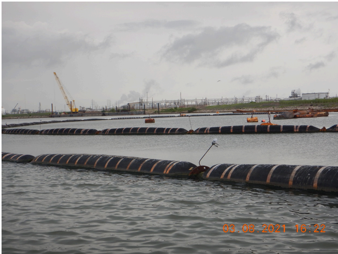
Figure 26: Photo of Floating Dredge Equipment
