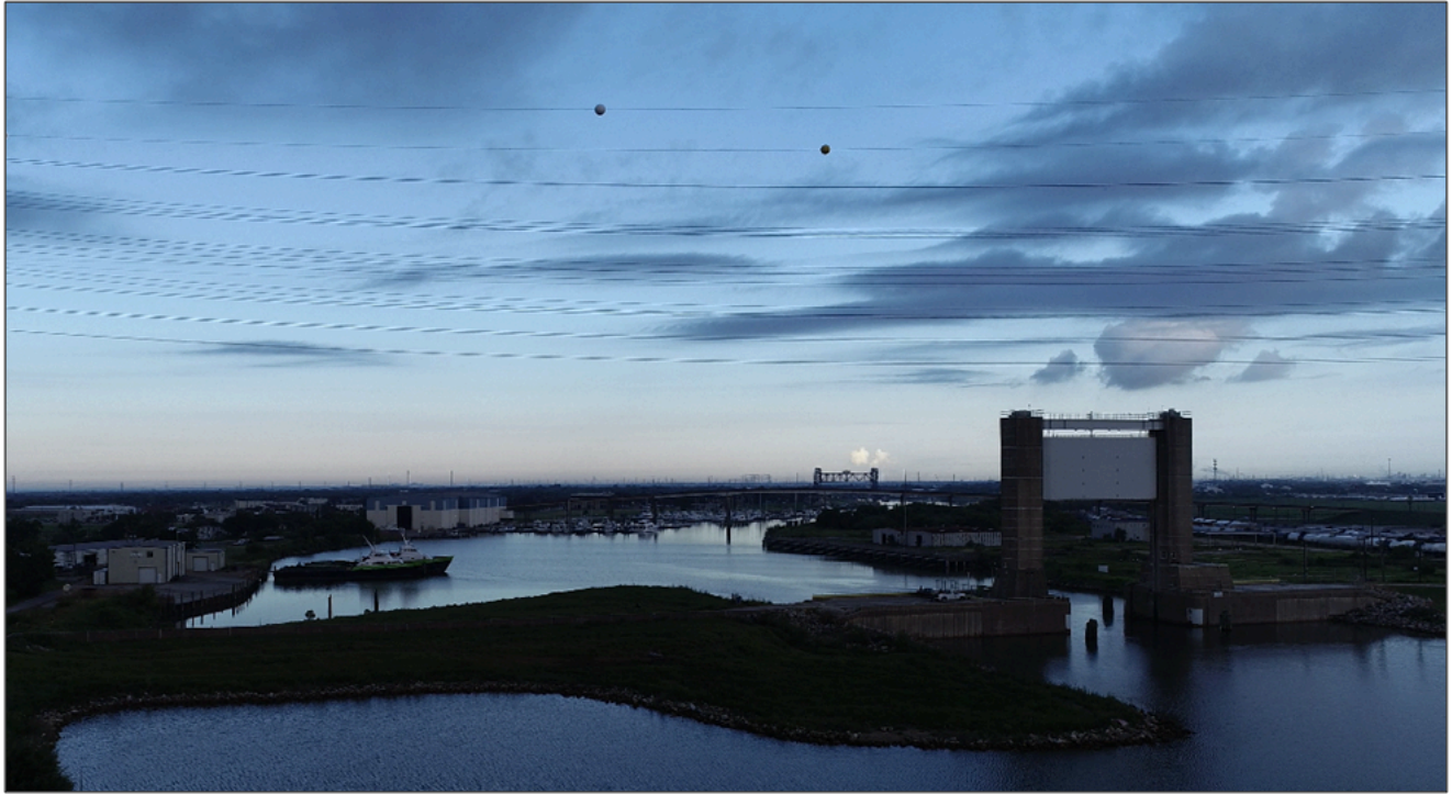
Figure 30: Tide Gate with Overhead Cable
