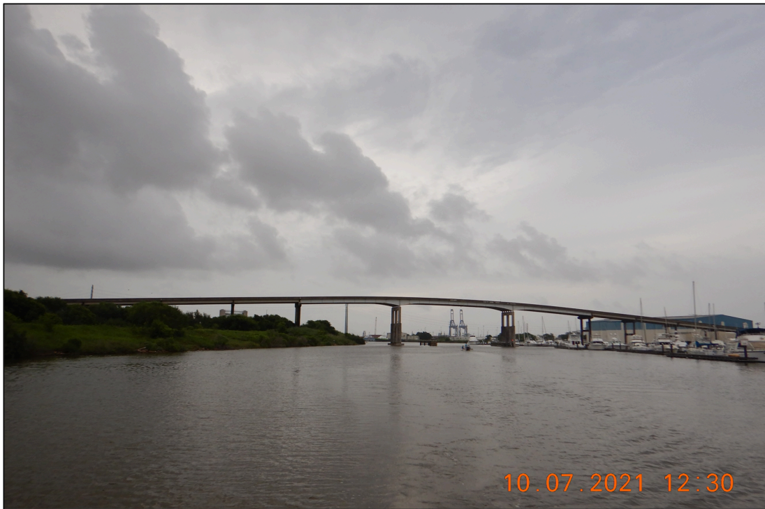
Figure 31: Pine Street Bridge
