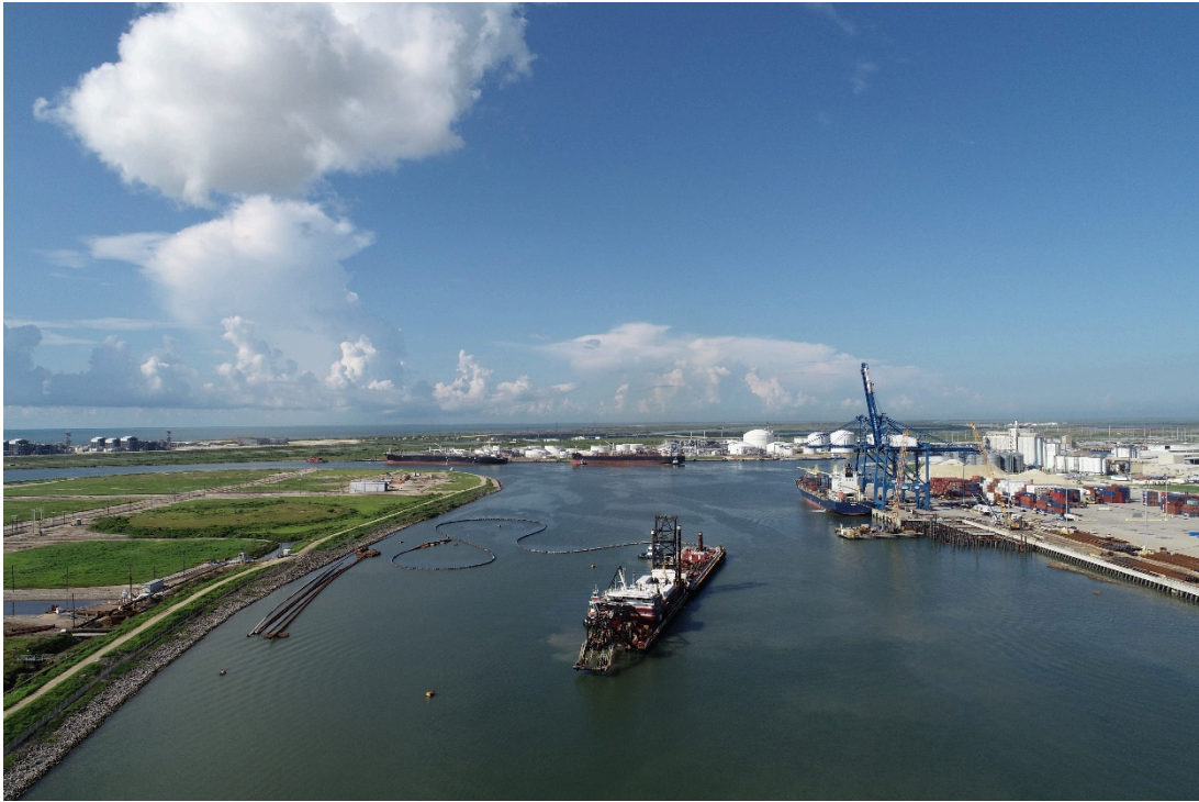
Figure 35: Overview of Primary Dredge Area
