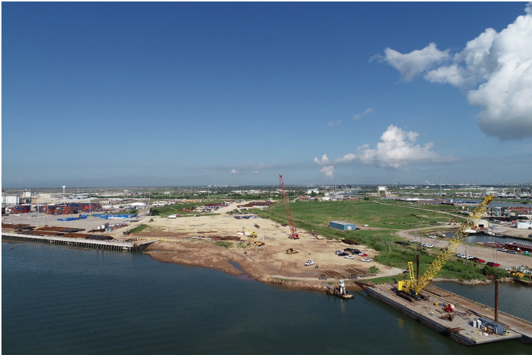
Figure 39: Active Construction at Port of Freeport, Photo 2
