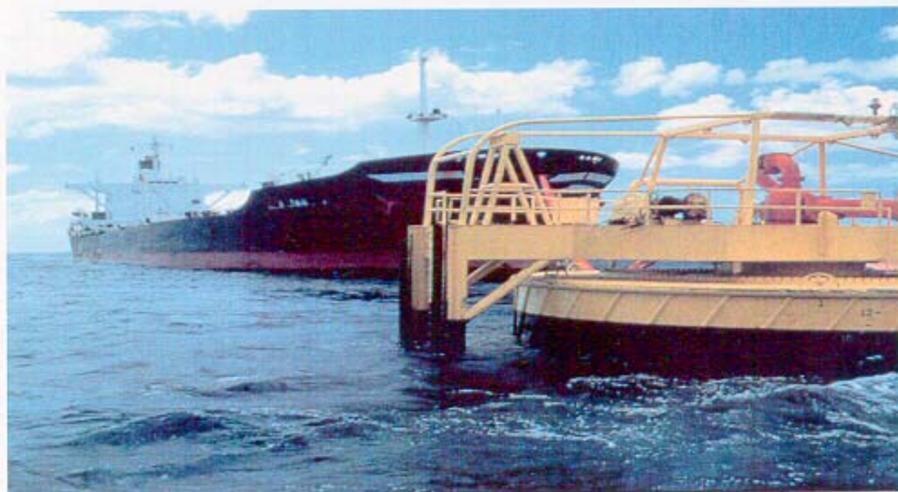
Figure 13. Barbers Pt, Oahu. Offshore oil terminal
