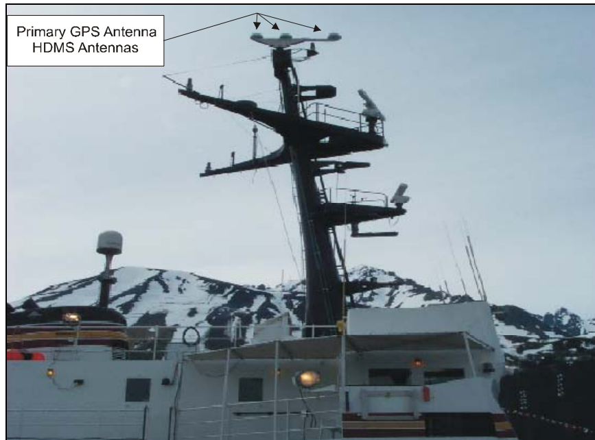
Figure B-4-1 Primary GPS and POS MV Antennas
