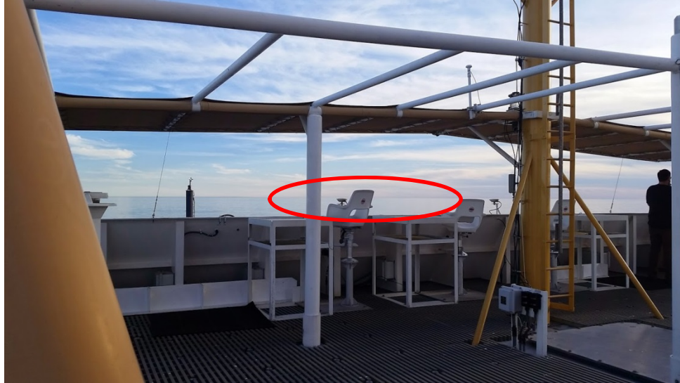
Figure 4: Image of POS antenna location on the flying bridge.
