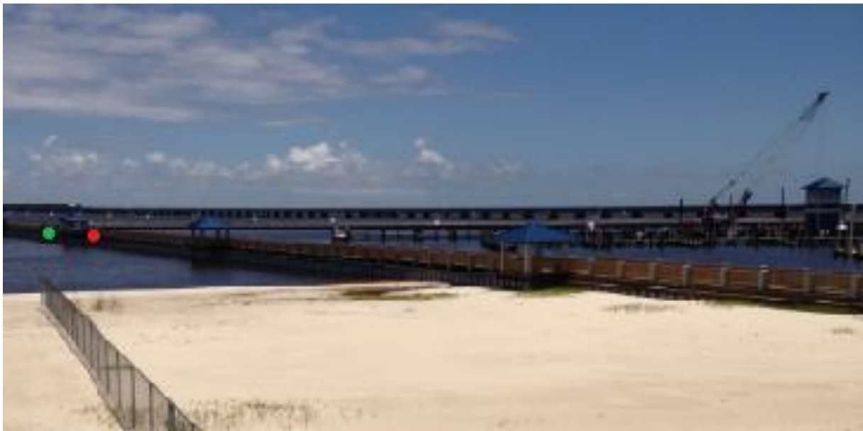
Figure A.4 View of the Jimmy Rutherford Fishing Pier.
