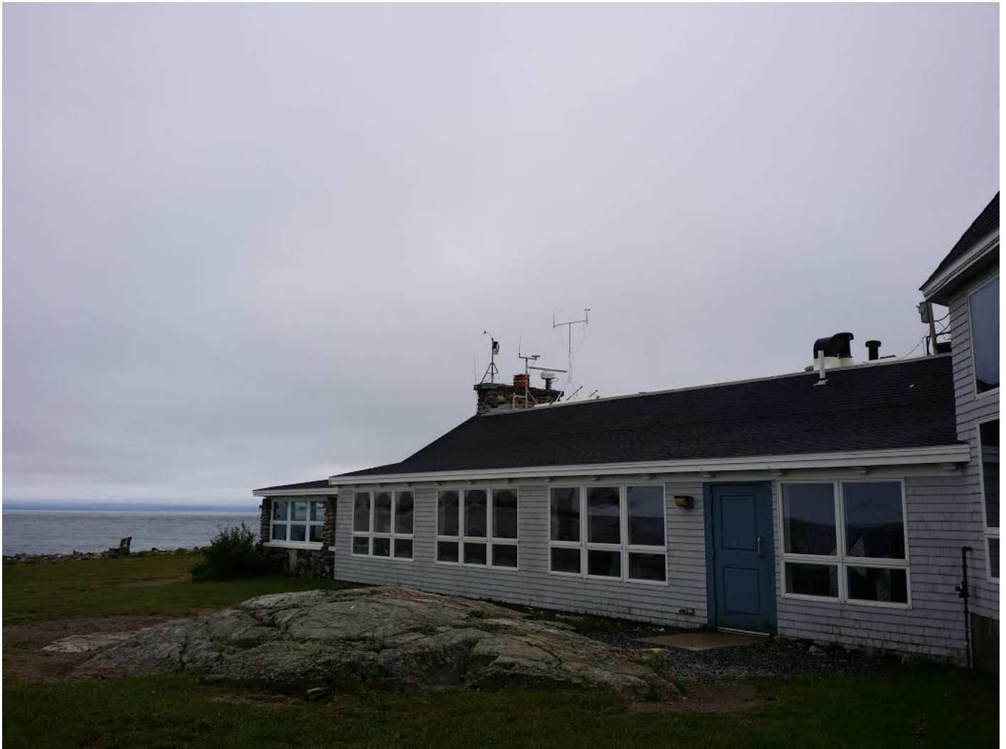
Figure 4: Odiorne RTK Base Station
