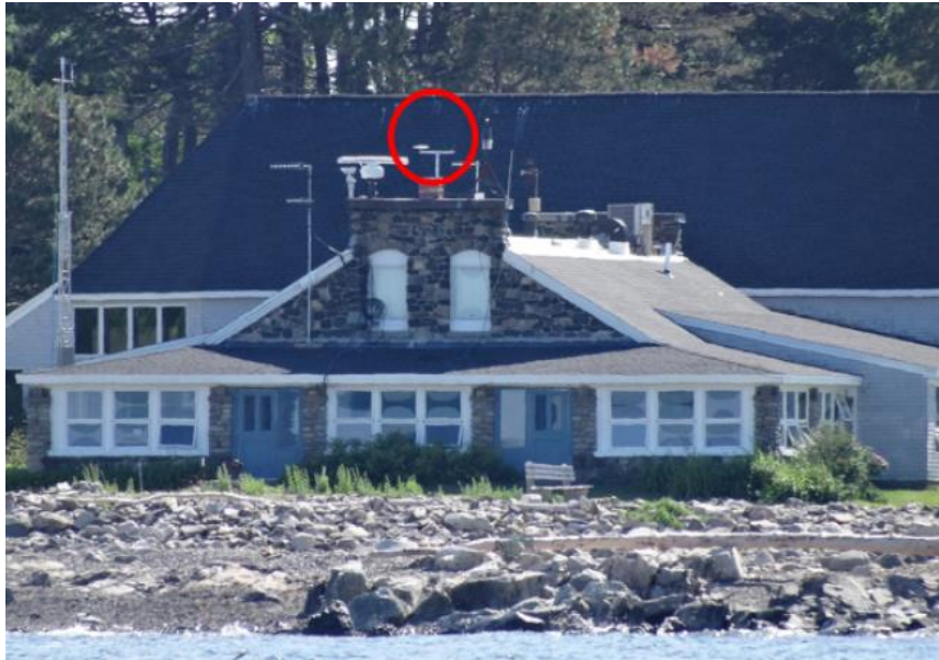
Figure 7. RTK base station at Odiorne Point.
