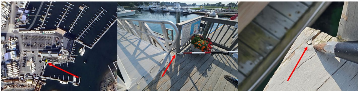
Figure 7. “CAM24-MLLW” is a nail in the decking adjacent to the northward metal gangway leading down to the docks at Cape Ann Marina in Gloucester, Massachusetts.
