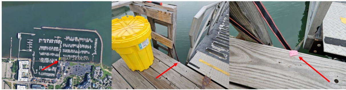
Figure 5. “MBAY 24 - MLLW” is a pink backed PK Nail in a dock at Safe Harbor Marina Bay in Quincy, Massachusetts.
